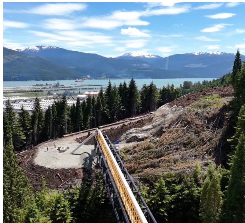
Completed pipeline, with restoration underway.
